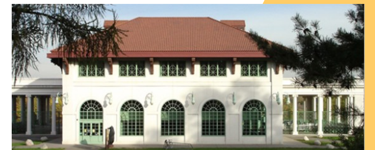
Como Lakeside Pavilion, future home of SML! Website: http://blackbearcrossings.com
